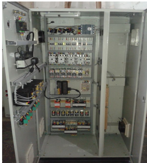
PLC CONTROL PANEL
