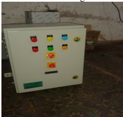
AHU.Control Panel
